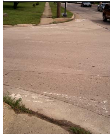
Deteriorated crosswalk striping
